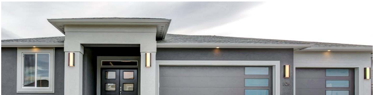
4" LED Wafers in Soffits
