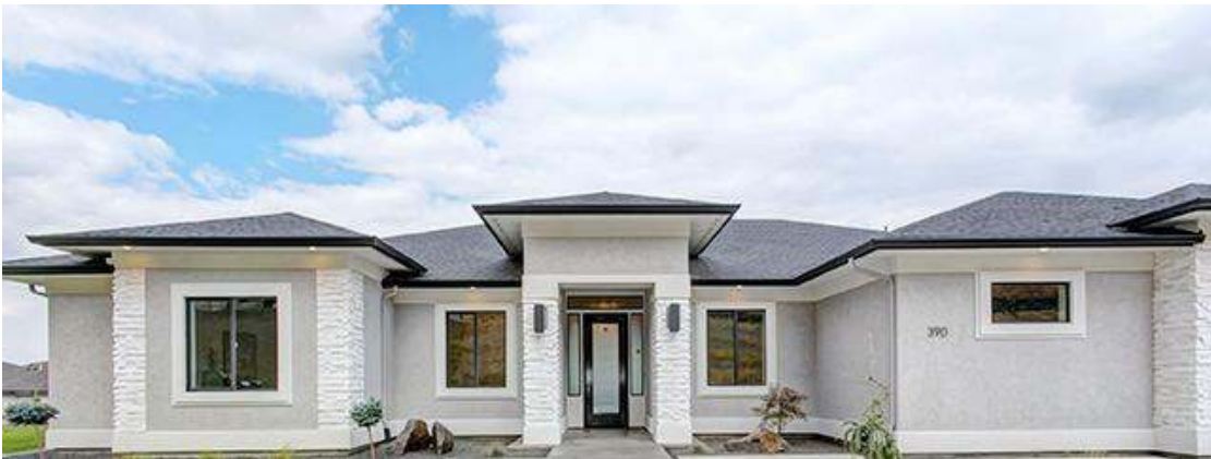
Base Trim & Soffit Trim at Front Elevation
