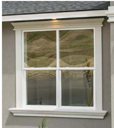
Sill and Skirt with Architrave Tops at Front Windows Only
