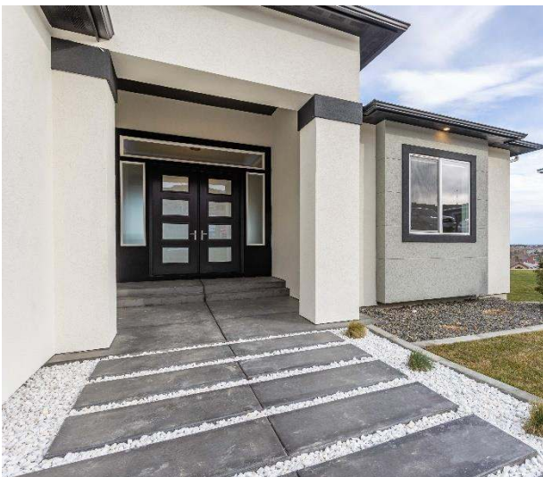
Modern Stacked, Broom Finish, Colored Concrete, Sealed, White China Rock. Extended.
