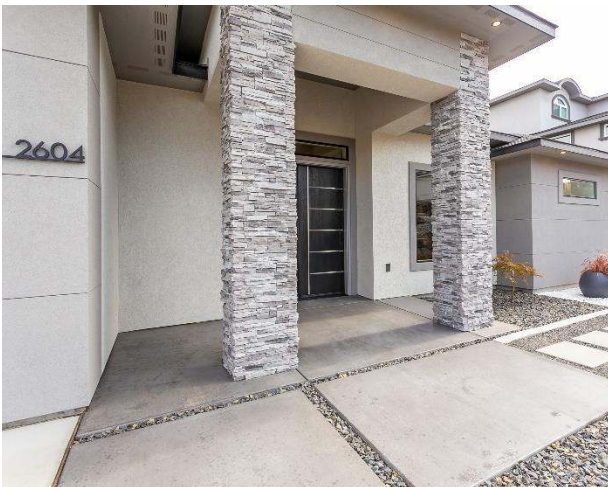
Modern Stacked, Broom Finish, Sealed (Not extended)
