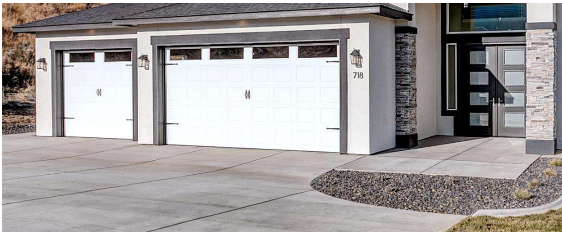
Broom Finished Driveway, Lead Walk, and Front Porch
