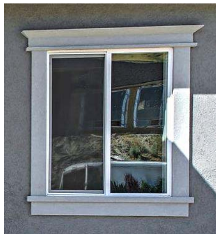
Sill and Skirt with Architrave Tops at Front Windows
