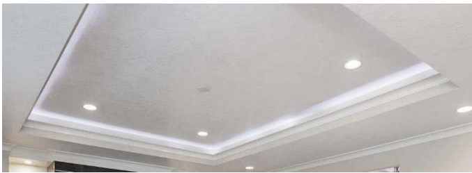
LED Rope Lighting in Tray Ceiling
