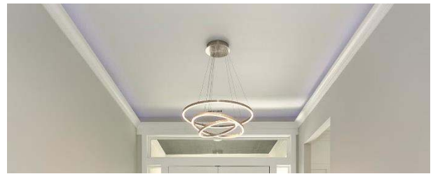
LED Rope Lighting in Dropped Crown
